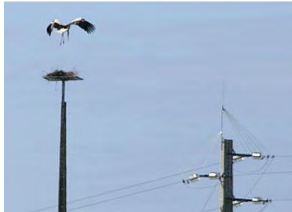
Figure 11. Distribution pole with symmetric chevron (arrow) on top as bird exclusion device (Photo: EDP-Distribution, Portugal; and distribution pole with bird exclusion spikes with dedicated nesting pole for White Stork next to it (Photo: Carlos Tiago).
