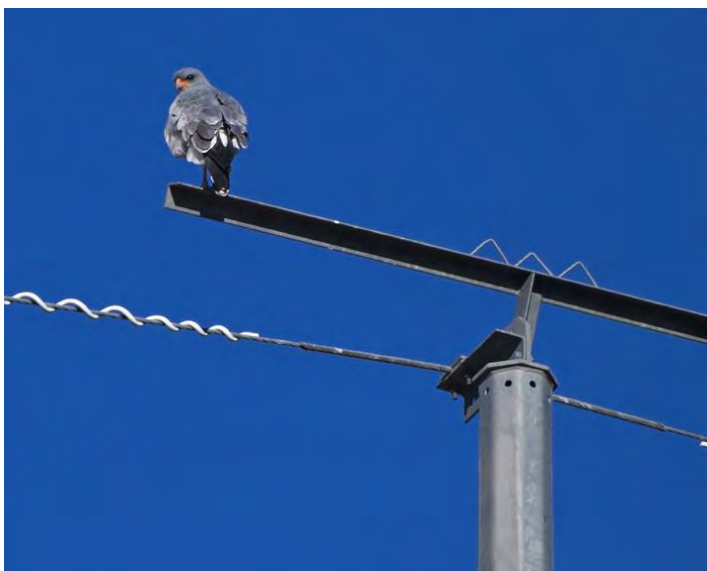
Figure 11. Distribution pole with symmetric chevron (arrow) on top as bird exclusion device (Photo: EDP-Distribution, Portugal; and distribution pole with bird exclusion spikes with dedicated nesting pole for White Stork next to it (Photo: Carlos Tiago).
