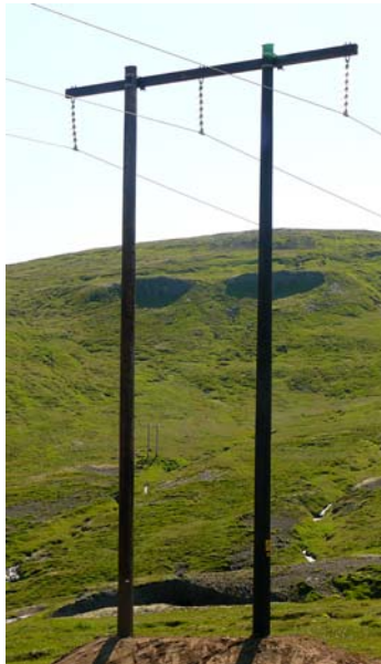
Figure 4. Left: a safe horizontal low voltage line, with three conductors suspended below cross-arm with sufficiently long insulators. Right: a low voltage line in Iceland unsafe for larger waders, here Whimbrel ( Numenius phaeopus ) and Black-tailed Godwit ( Limosa limosa islandica ) and larger raptors (in this case White-tailed Eagle ( Haliaeetus albicilla ) and Gyr Falcon ( Falco rusticolus )) because of conductors attached on short insulators on top of cross-arm. In this case retrofitting could include insulating the central conductor wire and/or covering the insulators (Photo: Bureau Waardenburg).
