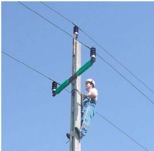
Figure 7. Cross-arm insulation carried out in Hungary (source: Horvath et al., 2011).
