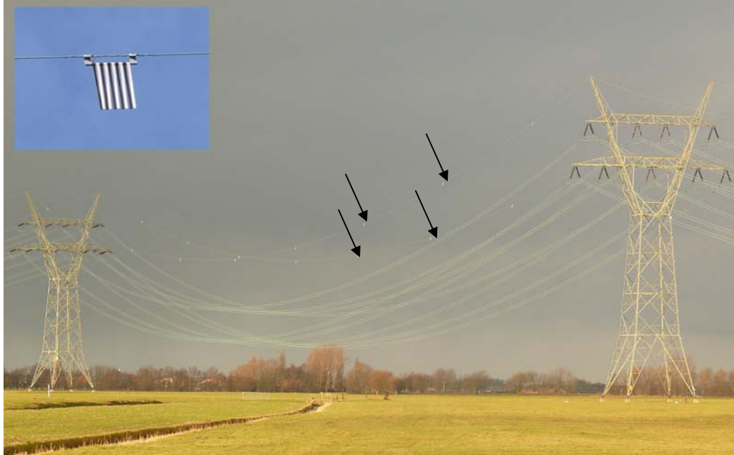
Figure 20. High tension (150 kV) power line in the Netherlands with bird flappers (see arrows) placed at regular intervals in both ground wires as bird flight diverters, see also Box 1 (Photo: Bureau Waardenburg).
