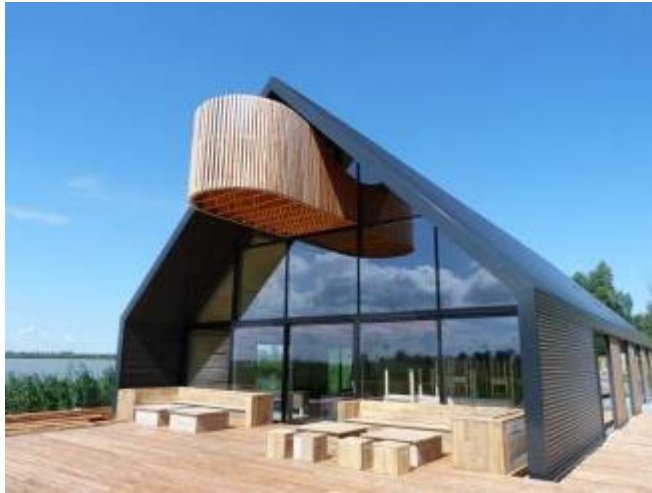
The present centre in the final stage of construction.
