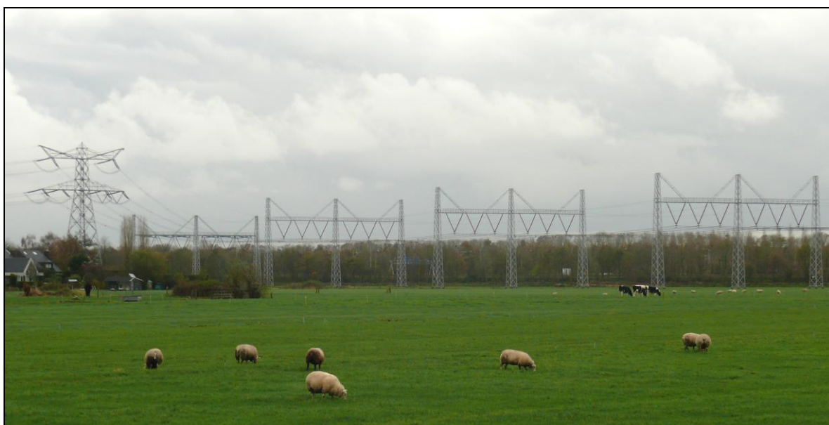
Figure 17: A 380 kV line, with lowered conductor wires hanging from portals in one horizontal plane to minimise collision risk for Great Cormorant ( Phalacrocorax carbo ), Eurasian Spoonbill ( Platalea leucorodia ) and Purple Heron ( Ardea purpurea ) daily passing this stretch of line while commuting between the breeding colony and foraging areas, Muiden, the Netherlands (Photo: Bureau Waardenburg).
