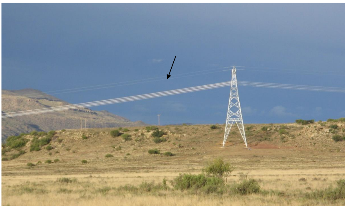
Figure 16: A 400 kV line, with all conductor wires in the same horizontal plane. This picture also demonstrates the almost invisible thin earth wire (black arrow) in top (Photo: EWT-WEP).
