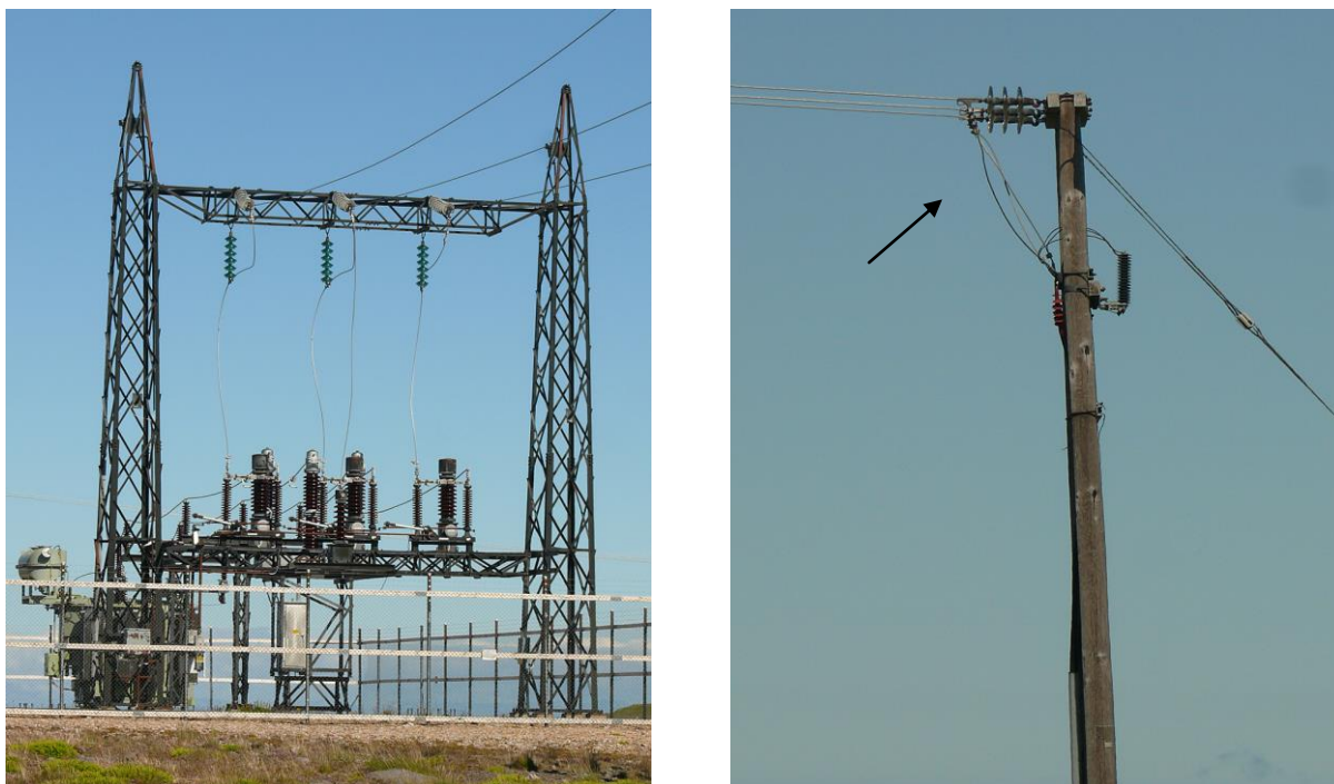
Figure 3: Left: Distribution substation with some closely spaced energised parts that is potentially dangerous to birds. Retrofitting could include insulation of vertical hanging wires and spatial separation of energised parts. Right: End pole of distribution line; jumper wires (arrow) are constructed below conductors and insulators are more than 60 cm long, providing a bird-safe perch on top of the pole (Photos: Bureau Waardenburg).
