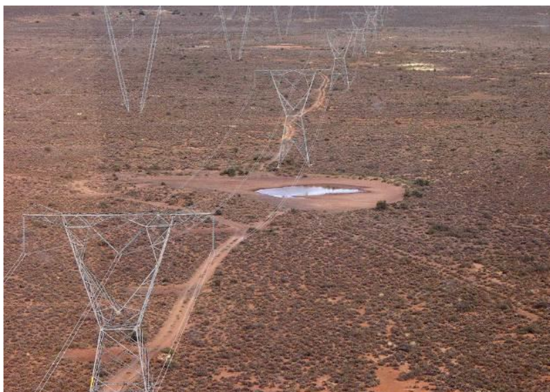
Figure 1: Two adjacent transmission lines in the Karoo region of South Africa. The sum of impacts on birds from two closely spaced lines may be significantly lower than from lines positioned far apart (Photo: EWT-WEP).
