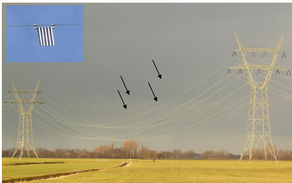
Figure 20: High tension (150 kV) power line in the Netherlands with bird flappers (see arrows) placed at regular intervals in both ground wires as bird flight diverters, see also Box 1 (Photo: Bureau Waardenburg).
