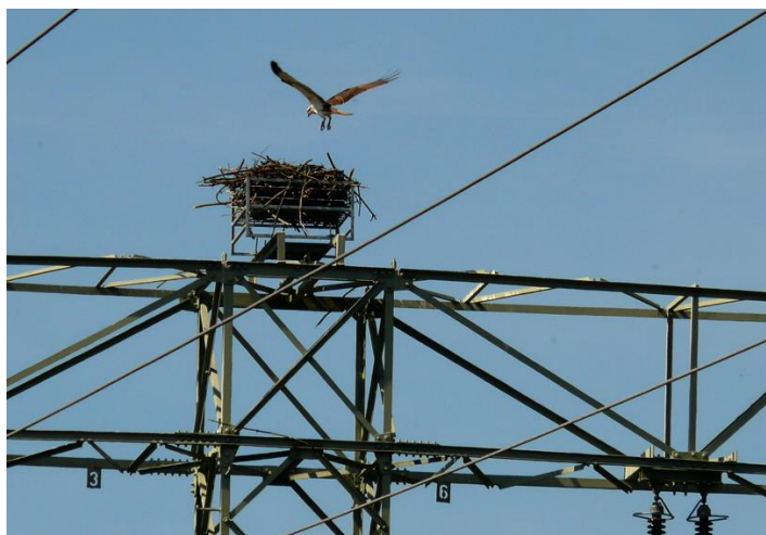
Figure 15: Nesting Osprey on artificial platform in medium voltage transmission line, Muritz National Park, Germany (Photo; Bureau Waardenburg).
