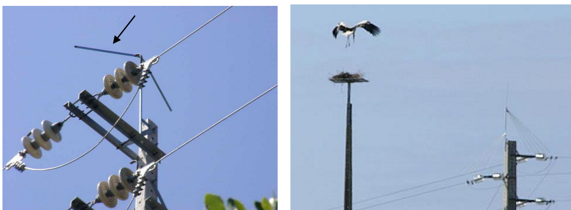
Figure 11: Distribution pole with symmetric chevron (arrow) on top as bird exclusion device (Photo: EDP-Distribution, Portugal; and distribution pole with bird exclusion spikes with dedicated nesting pole for White Stork next to it (Photo: Carlos Tiago).
